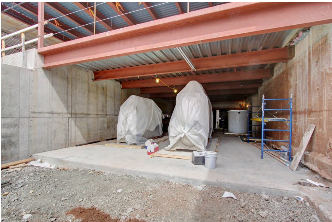
Mechanical equipment is installed in the new chiller room beneath what will be a new Biology CLAB (Classroom/Lab Combination) above. Monday, April 14, 2014
