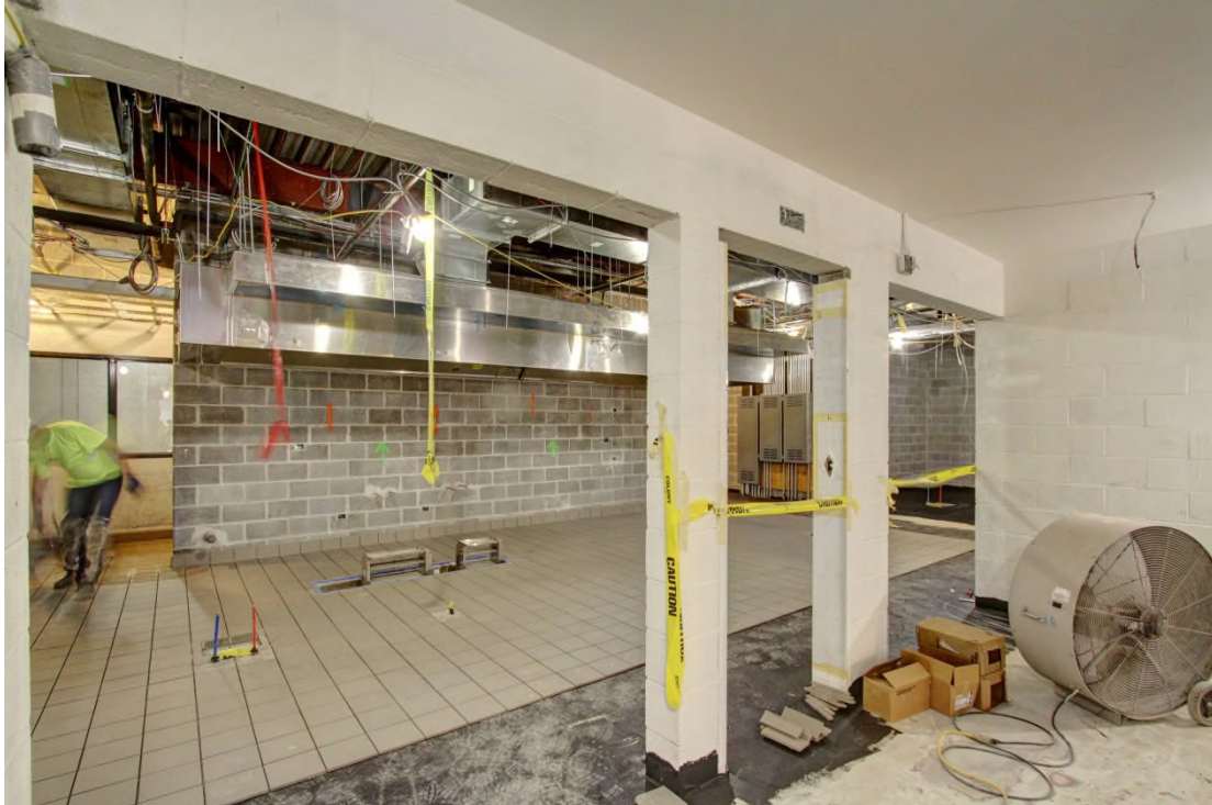
Waterproofing membrane and quarry tile being installed in the kitchen prep area. Monday, April 14, 2014
