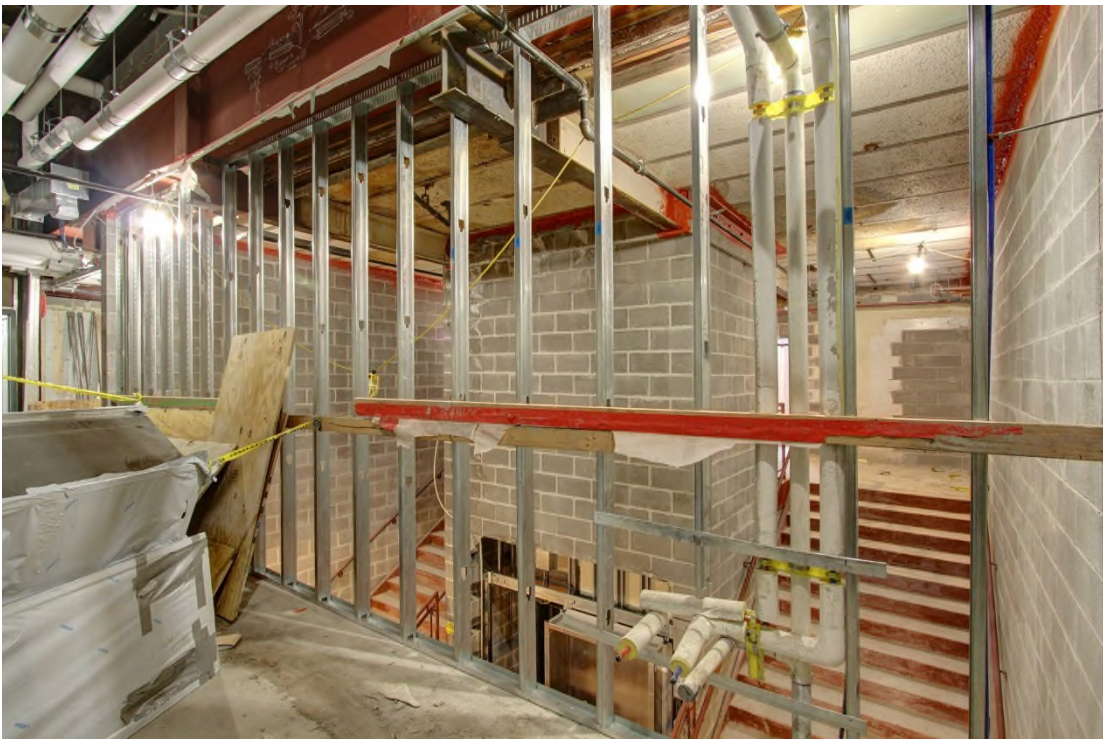
The new wall is framed separating the science storage from the new elevator and twin stairs to the lower level. Wednesday, April 23, 2014
