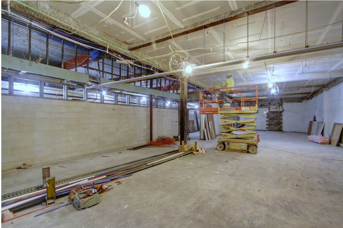
Overhead rough-in continues in new Social Studies classrooms. This space will be flexible with a movable partition supported on a track above the ceiling.
