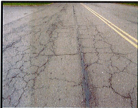
Christian Lane – North of Deming Road Longitudinal and Alligator Cracking
