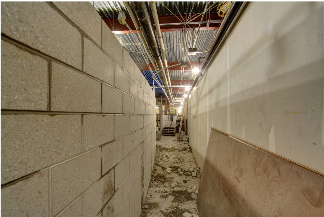
A view of the new curved ground face block from the corridor side of the walls. Tuesday, February 25, 2014
