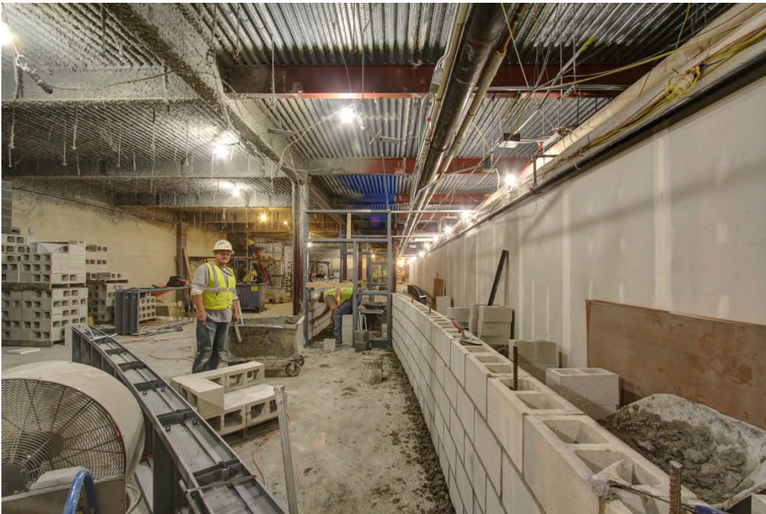
The new curved masonry walls built from ground face block continue to take shape. These walls will form the separation between new social studies classrooms and the corridor where the new light-well will be cut into the floor above.
