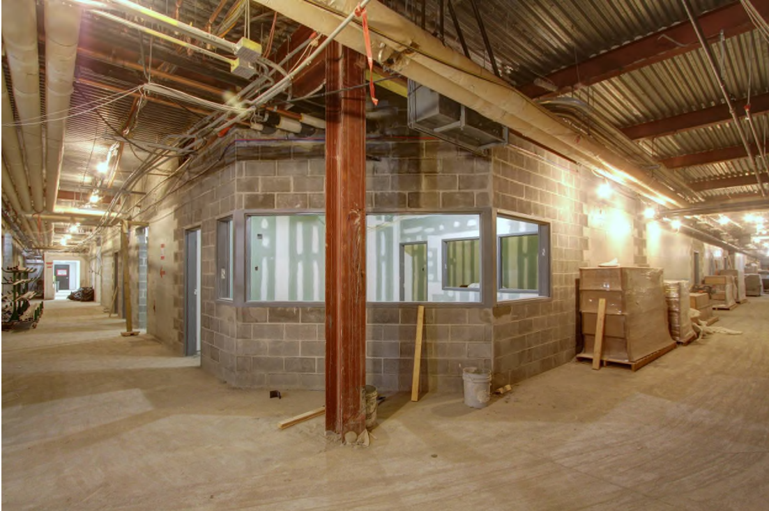
The radio station walls are complete and ready for primer and final paint. Friday, February 21, 2014
