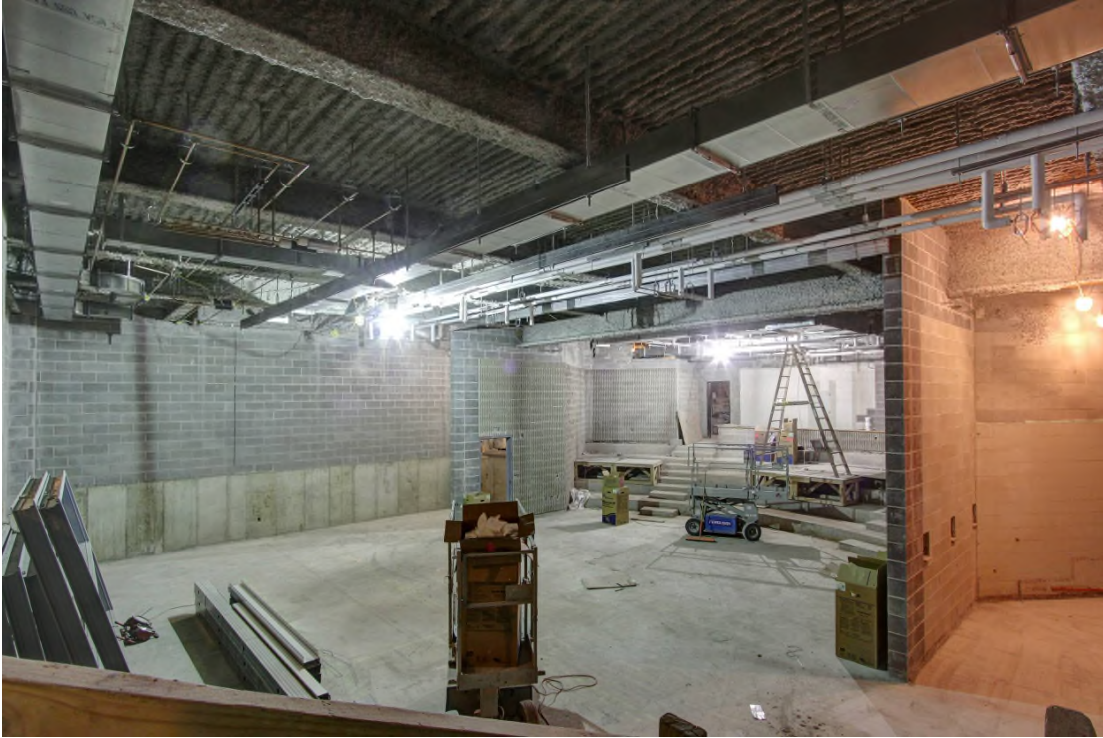
The new masonry wing walls pictured earlier are completed in the amphitheater and the new TV Studio.
