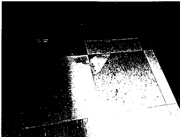
Figure 6. Damaged section of VCT flooring with adhesive layer exposed.
