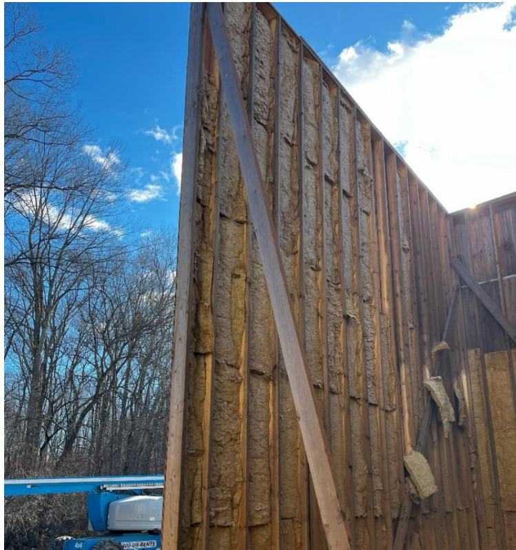
Figure 1: Exterior Exhaust 2-Sided Barrier
