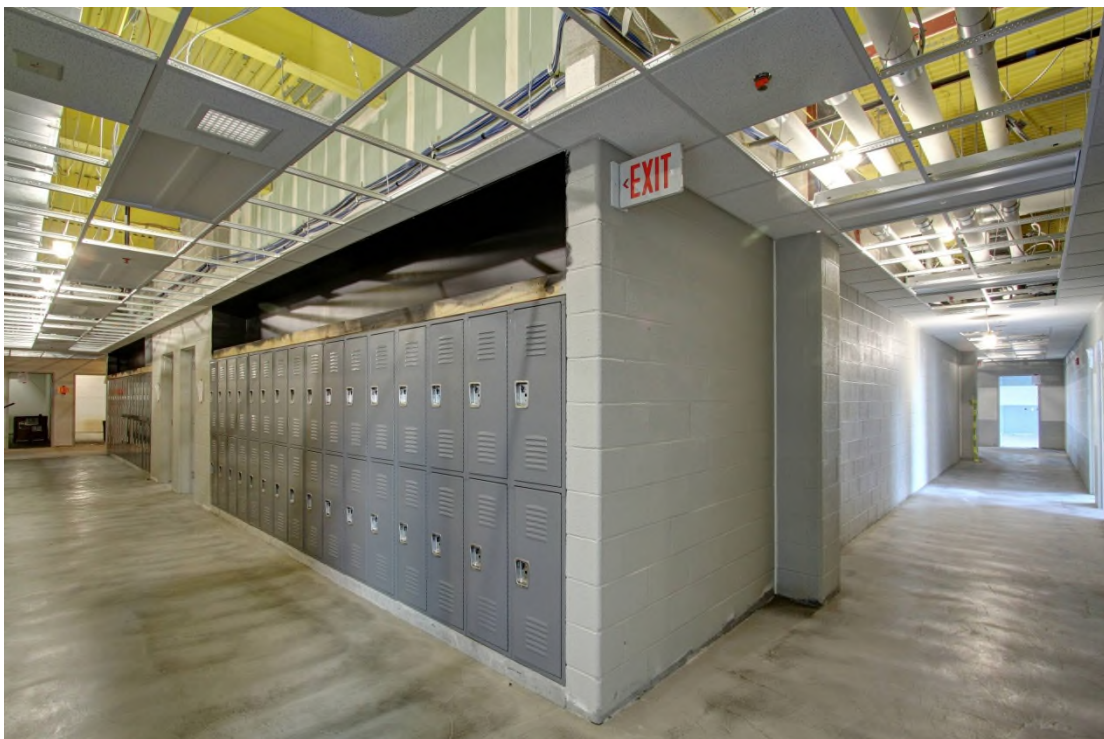
English wing hallways are prepped with lockers installed and the floor prepped for tile and base. Tuesday, May 6, 2014
