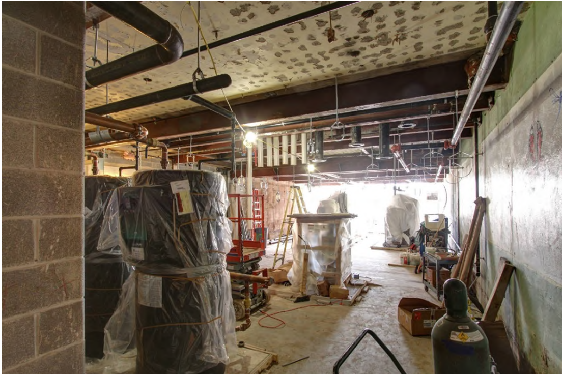
The new chiller room is loaded with equipment and piping work has begun. Friday, May 2, 2014
