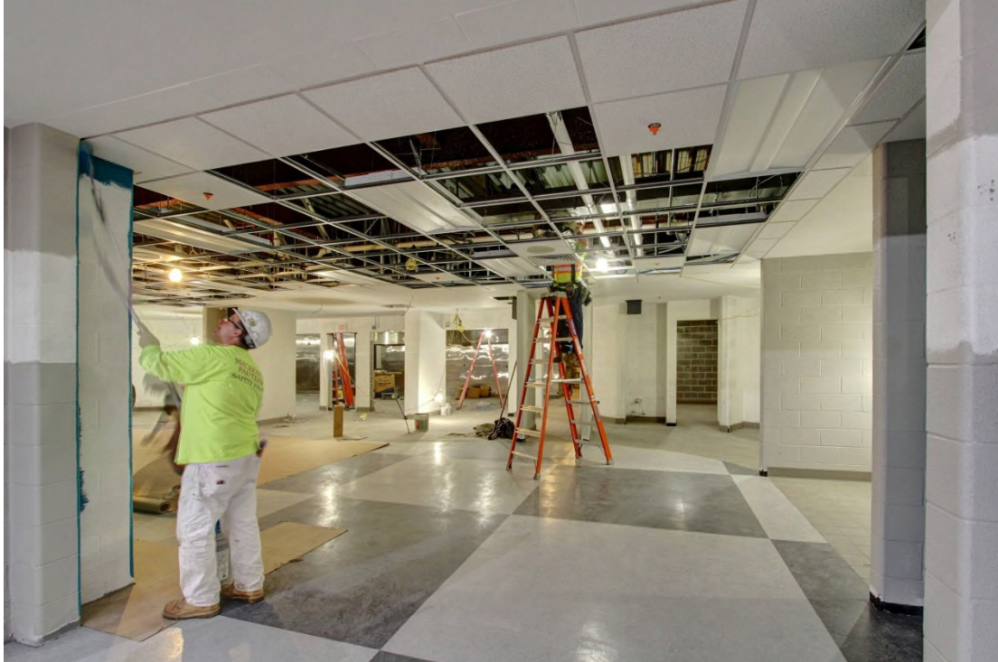
The new floor tile running from the cafeteria into the server ends when it meets the quarry tile under the new serving line.
