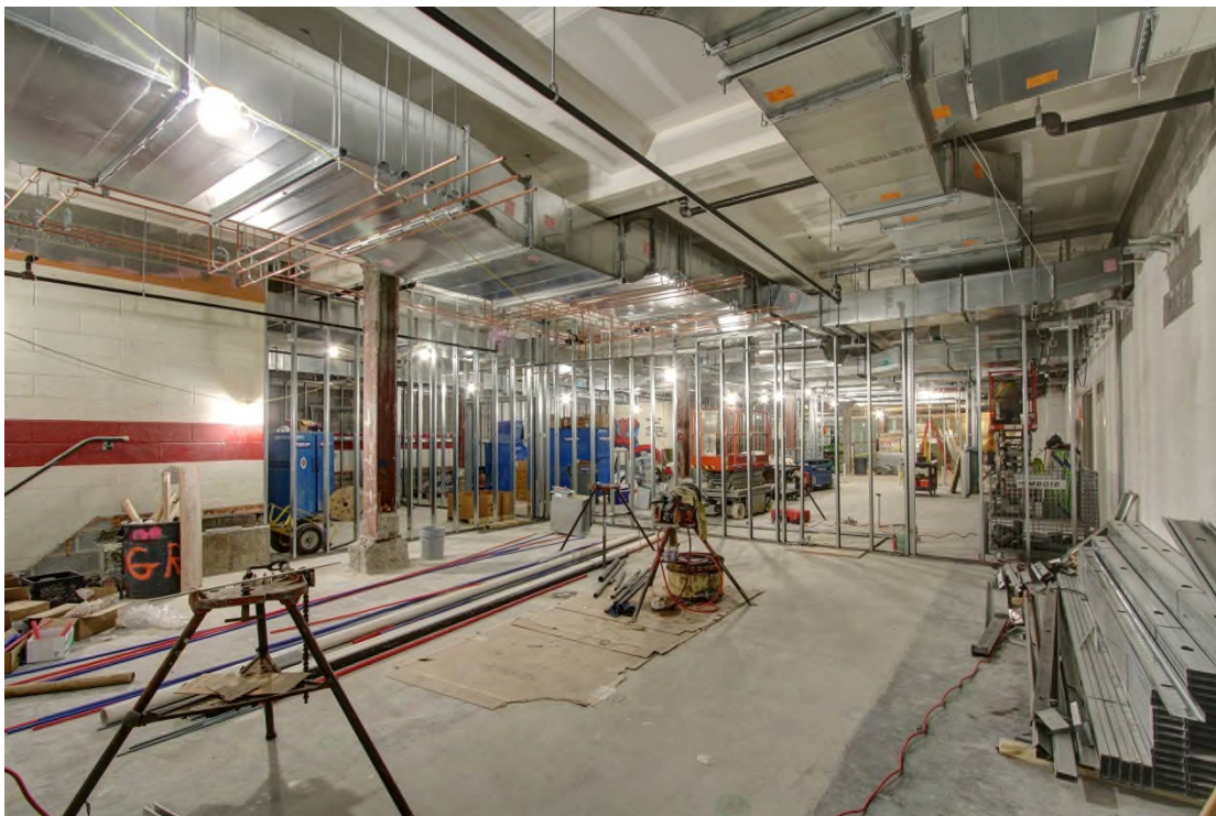
Overhead mechanical, plumbing, and electrical work continues in a health classroom adjacent to the F&CS area under the main gym. Tuesday, May 6, 2014
